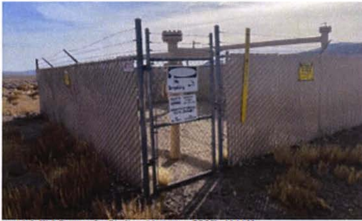
Photograph 3: High Pressure Gas Pipeline with transects PPOU - 12/14/23
