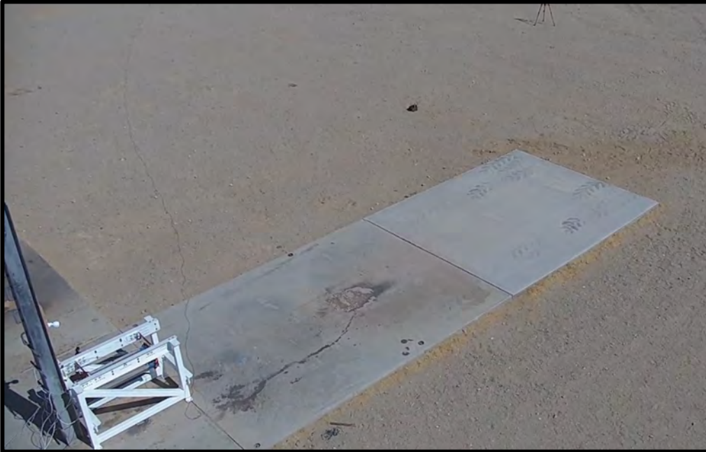
Test Pad (Churchill version will include sound berm)
