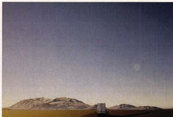
Visibility of Battery Storage Facility off Highway 50
