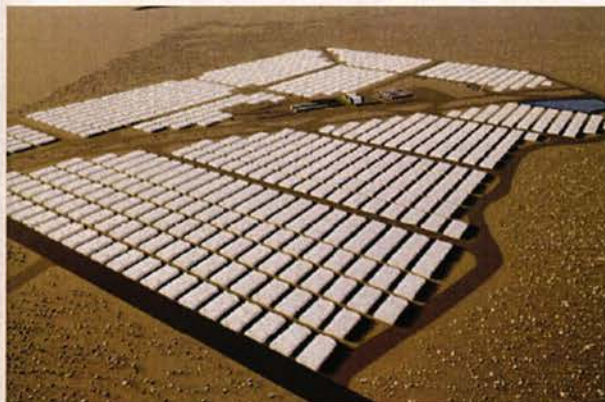
Overhead View of Battery Storage Facility
