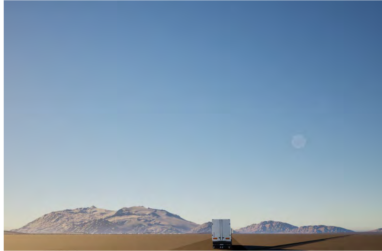
Visibility of Battery Storage Facility off Highway 50
