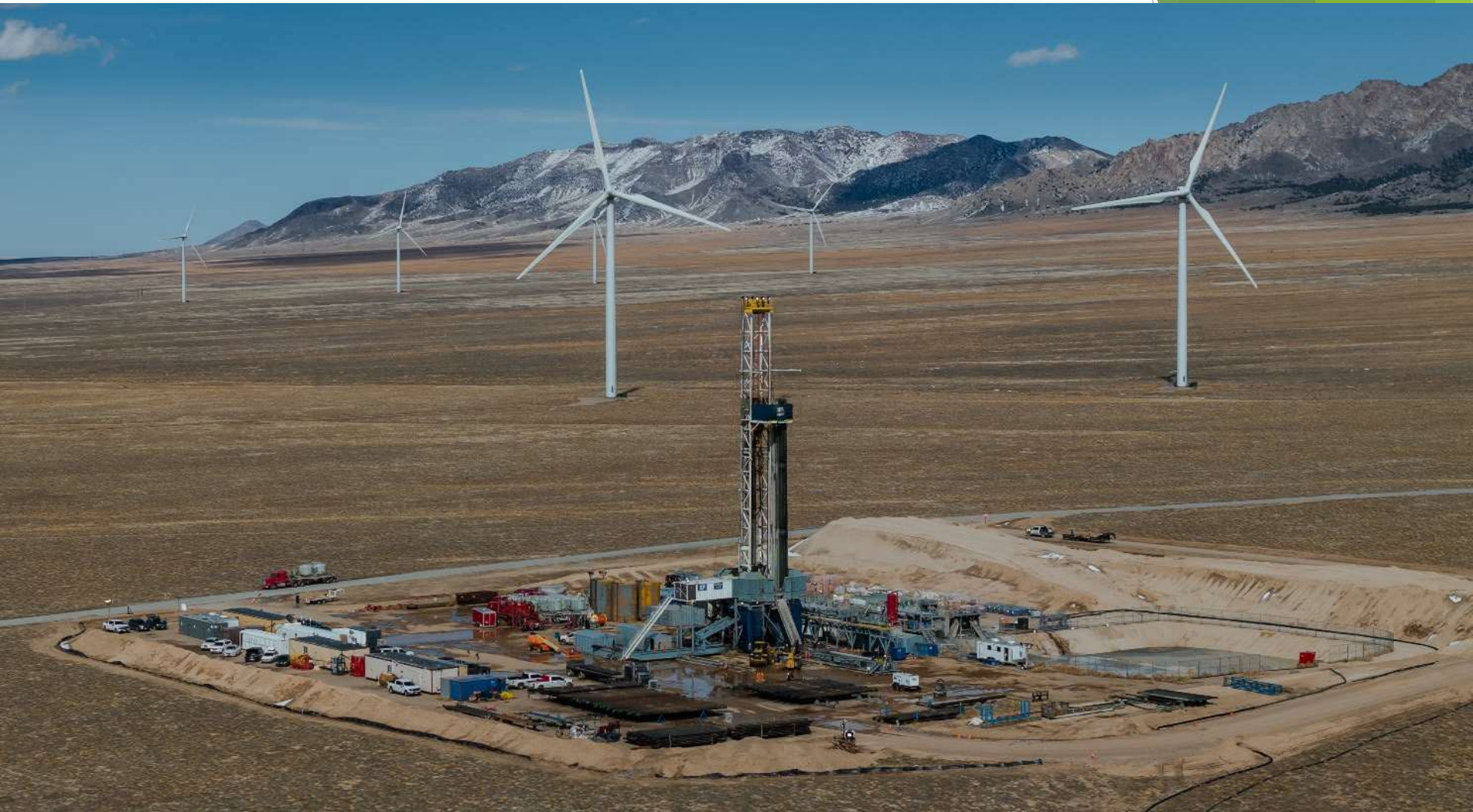
Well pad undergoing geothermal well drilling at the Cape Project in Utah
